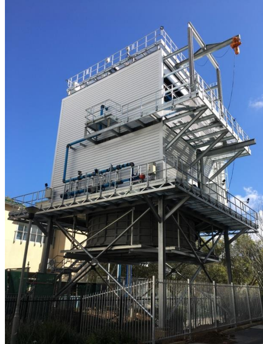
Photo: Full scale test facility nearly completed. Visible is the fan casing at the bottom as well as the deluge test section (opening at the top) (© ENEXIO Management GmbH, Kelvion Thermal Solutions (Pty) Ltd, Stellenbosch University).
